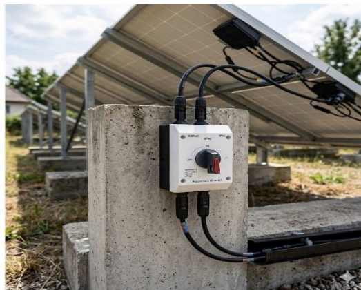
Figure 4.6: DC disconnect switch
