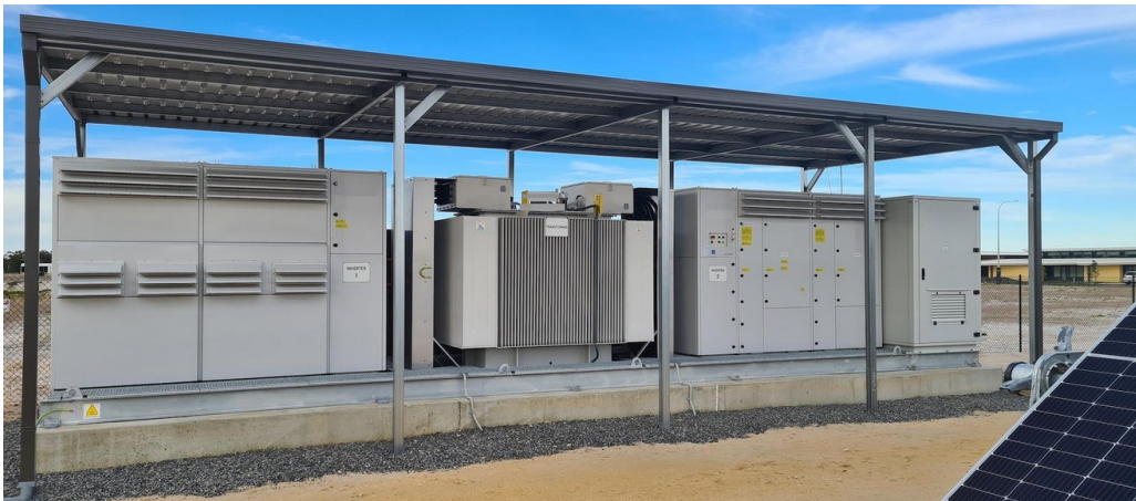
Figure 3.13: Inverter station
